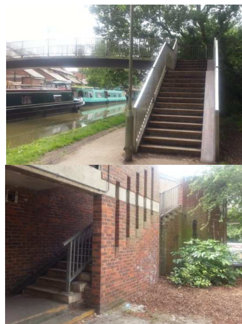
The existing footbridge to the north of the site
