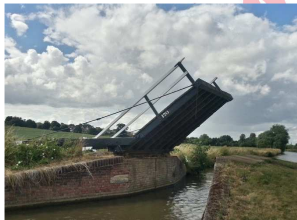
An example of a lifting bridge on the Oxford Canal
